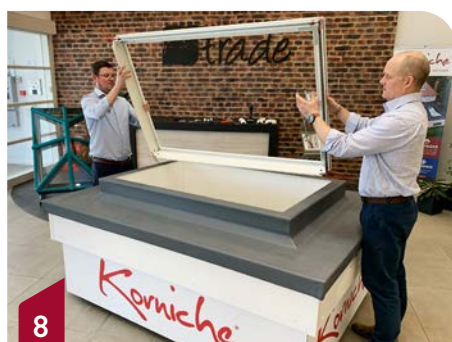
8 Carefully turn the connected eaves beams upside down ready to apply sealant to the underside of the assembly.
