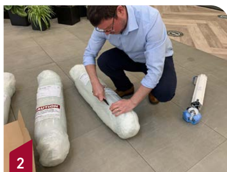
2 Always use a safety blade to unpack the parts to avoid scratching the profile surfaces.
