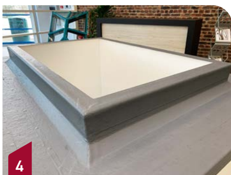
4 Ensure the prepared roof upstand is flat, dry and free of any debris. MFT advise a minimum of 150mm high and 69mm in width, providing t right base for the eaves beam of the lantern to be fixed down to.
