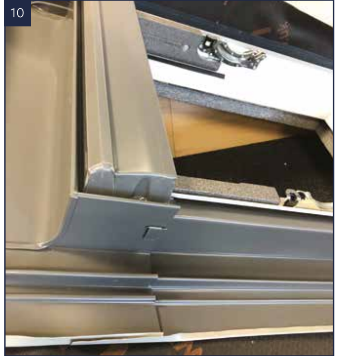
10 Position top section of flashing kit.
