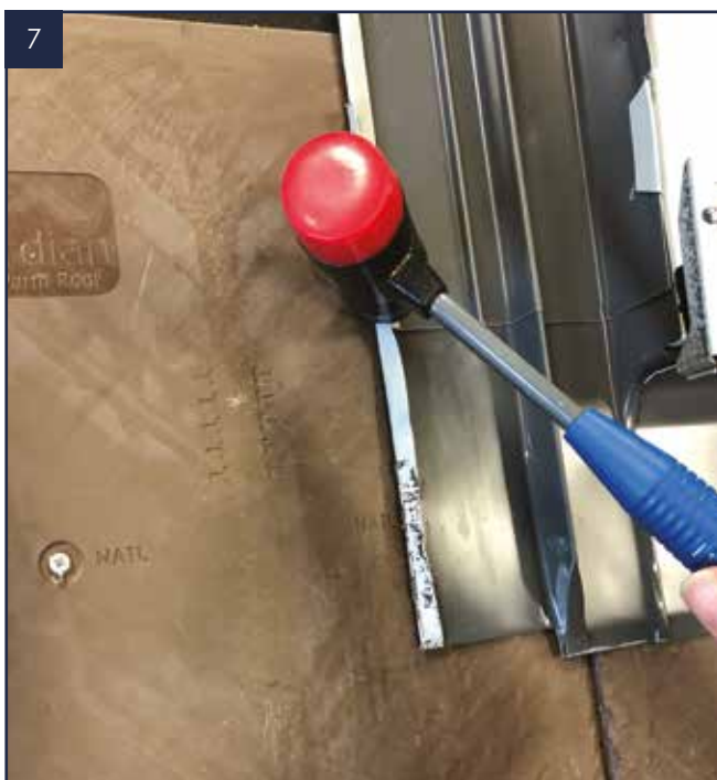
Fold over raised edge of the flashing kit using a plastic mallet or a hammer and block of timber.
