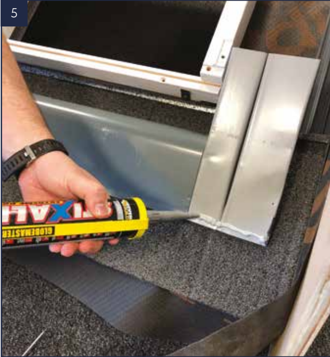
5 Nail tabs supplied in VELUX® flashing kit to the base of the frame, apply silicone to the underside and bottom edge of the flashing kit.
