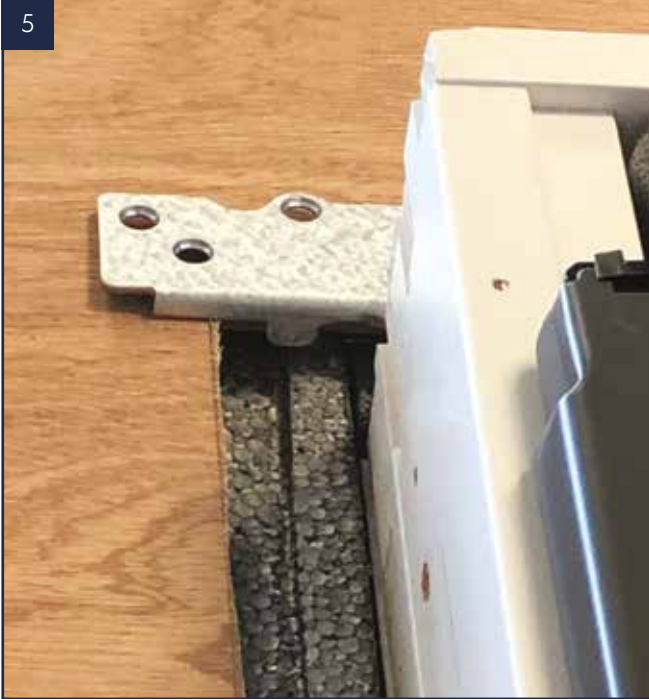
5 Check that the brackets are located at the top and bottom, and the frame is square.
