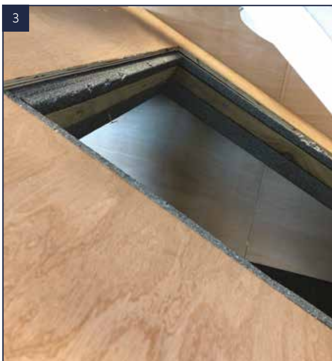
3 Ensure foam is fitted around aperture.
