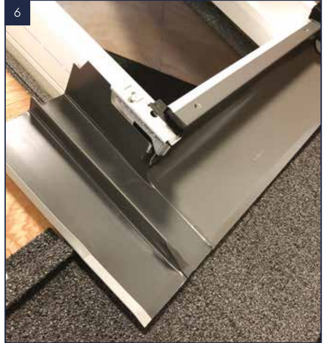
6 Sit the flashing in position and fold the tabs over to secure it.
