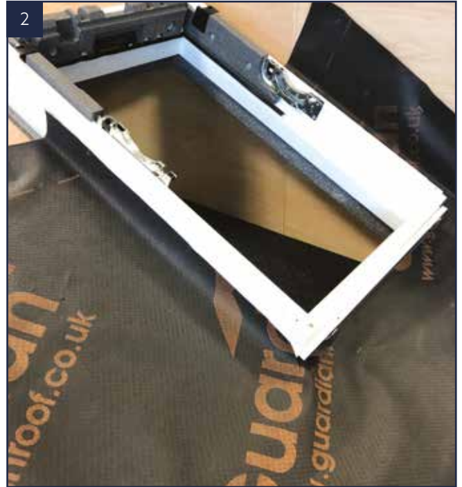
2 Lay the membrane on the roof and around the VELUX®.
