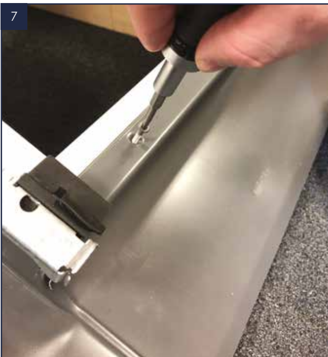
7 Fix the kit into the VELUX® unit using the screws provided.
