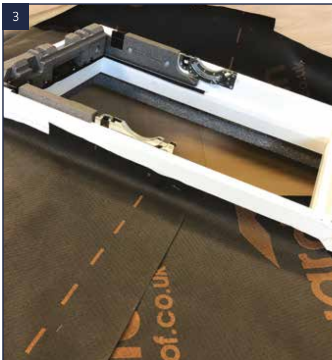
3 Ensure you leave a vertical lap all around the VELUX®.
