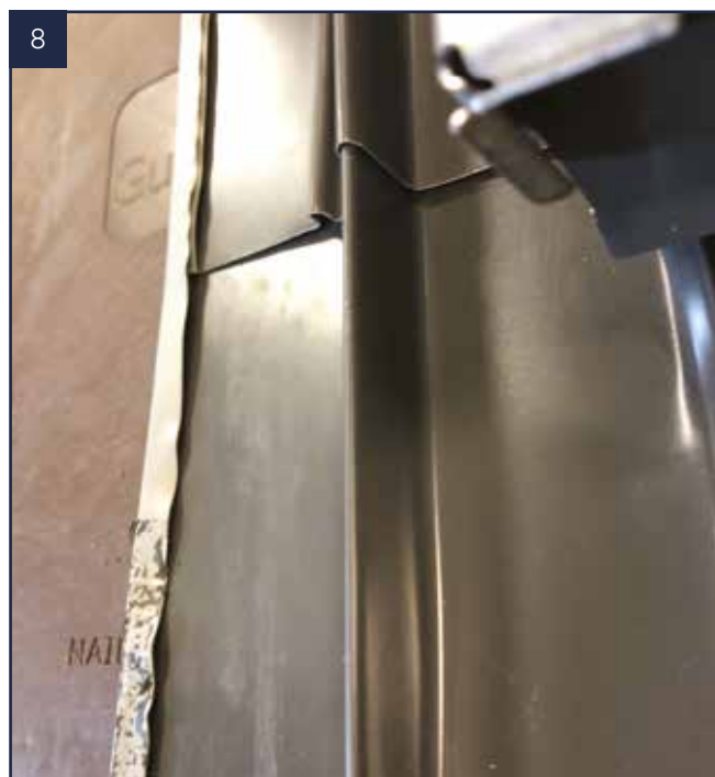
Try to get it as flat as possible so that the tiles can sit flush.
