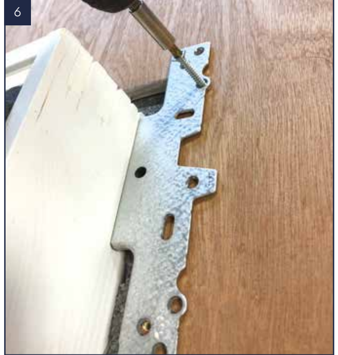
6 Once unit is centralised, secure to the roof using the fixing screws.
