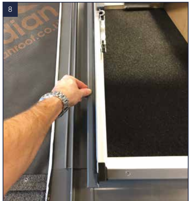
8 Position the side flashing parts .
