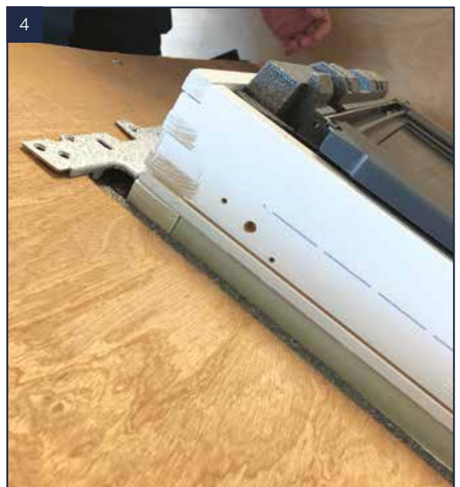
4 Align the unit central to the hole.
