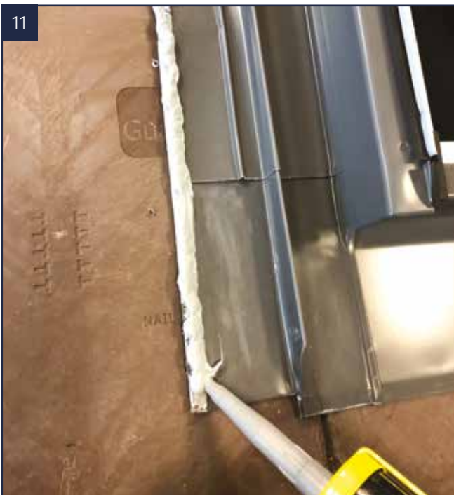
11 Run a bead of silicone down the flattened edge of the flashing kit where the next row of tiles will be fitting.
