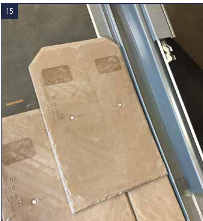
15 Continue sealing and fitting the rest of the slates in the standard pattern.
