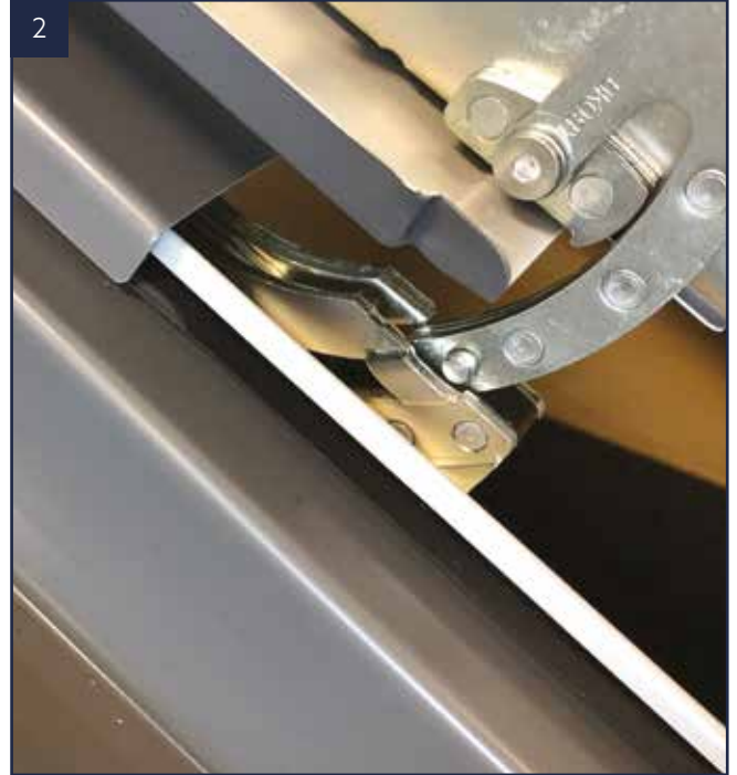
Engage the hinges and allow it to slot in. Then flip the sash over into the main frame.
