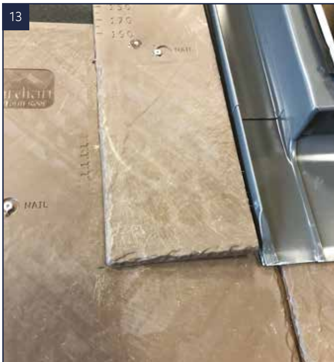
13 Press down in to place and screw down using fixings supplied.
