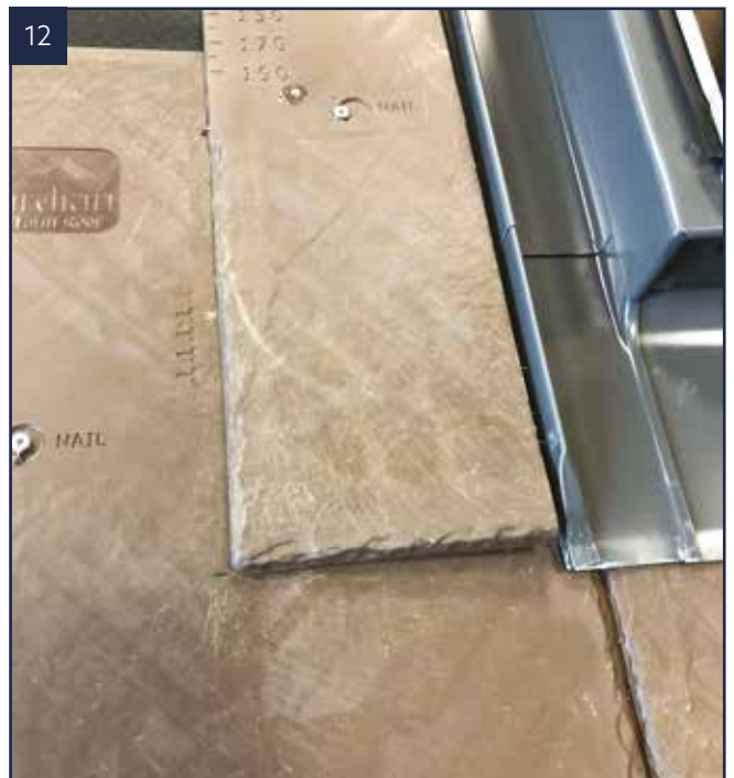
12 Position the first slate in line with the newly notched bottom edge of the kit.
