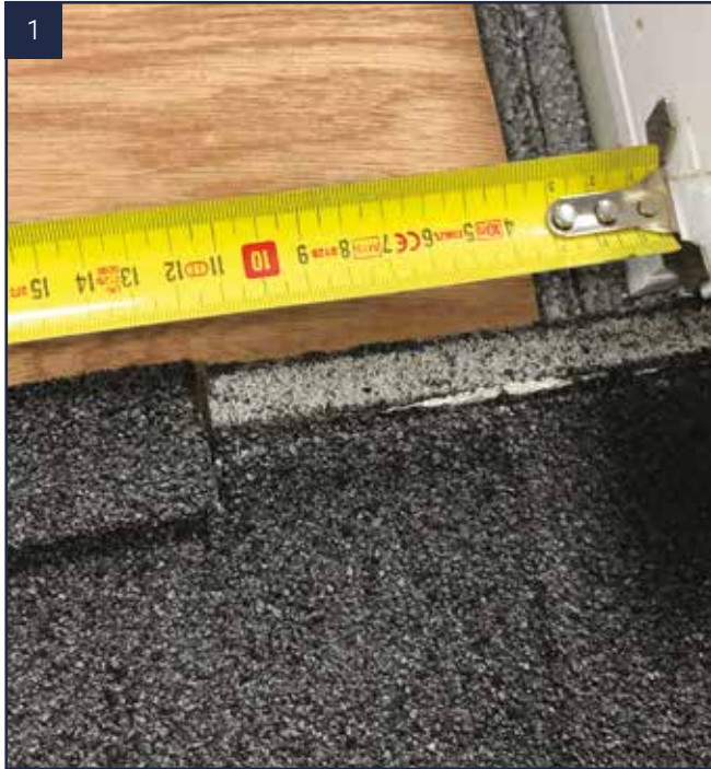
1 Pre-notch the lower tiles 120 mm either side of the VELUX® unit.
