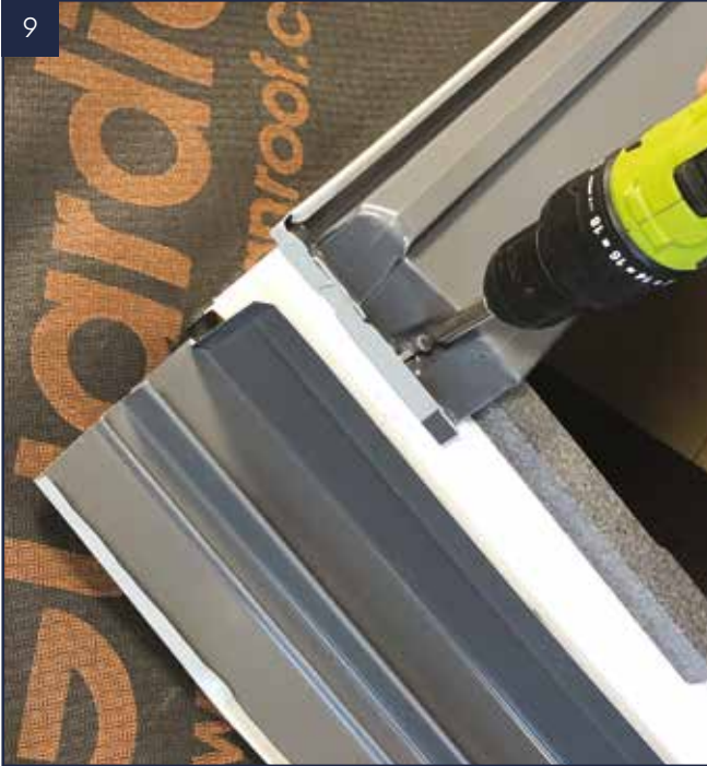
9 Fit top cover of the flashing kit and screw into place using fixings supplied.
