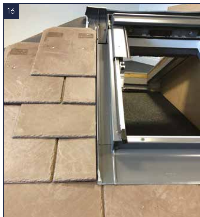
16 The finished tile edge and flashing kit should look as above.
