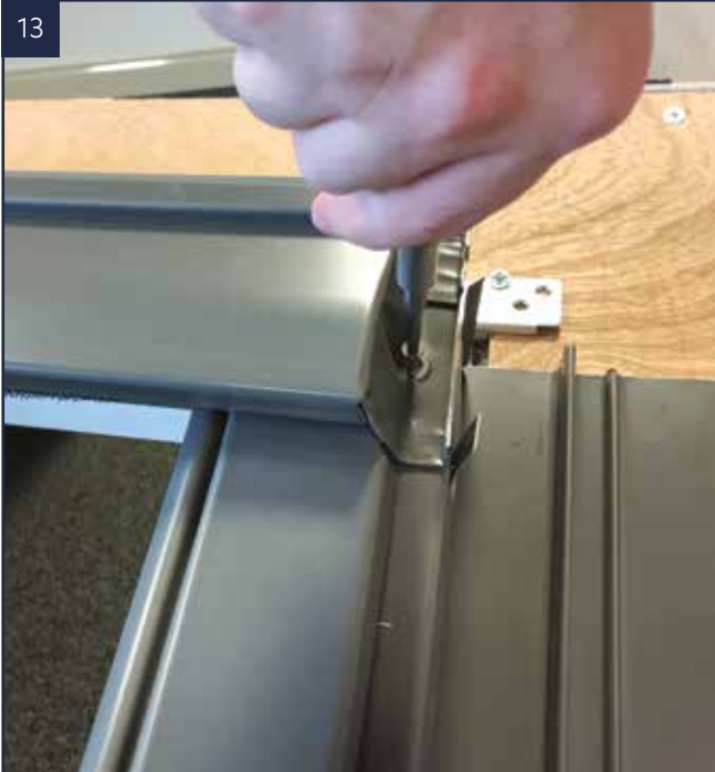
Fit top cover of the flashing kit and screw into place using fixings supplied.
