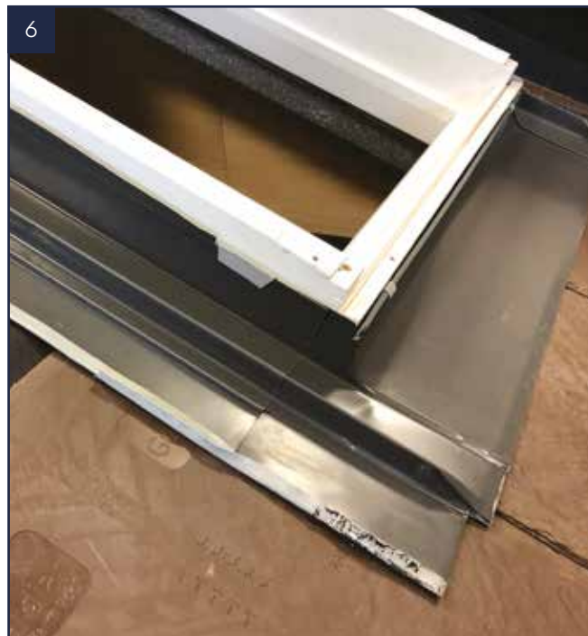
Position side flashing parts and fold over tabs.
