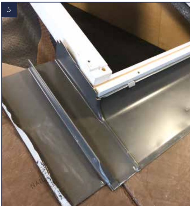
Sit the flashing kit into position, again pressing down to create a good seal to the slates.
