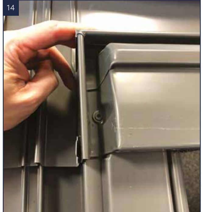
Slide down into place to create a tight fit slot over the top.
