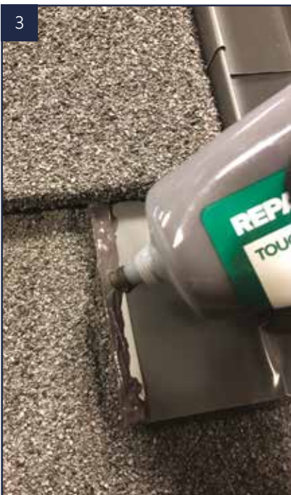
Use the touch up glue and grit to finish the bottom edge of the flashing.
