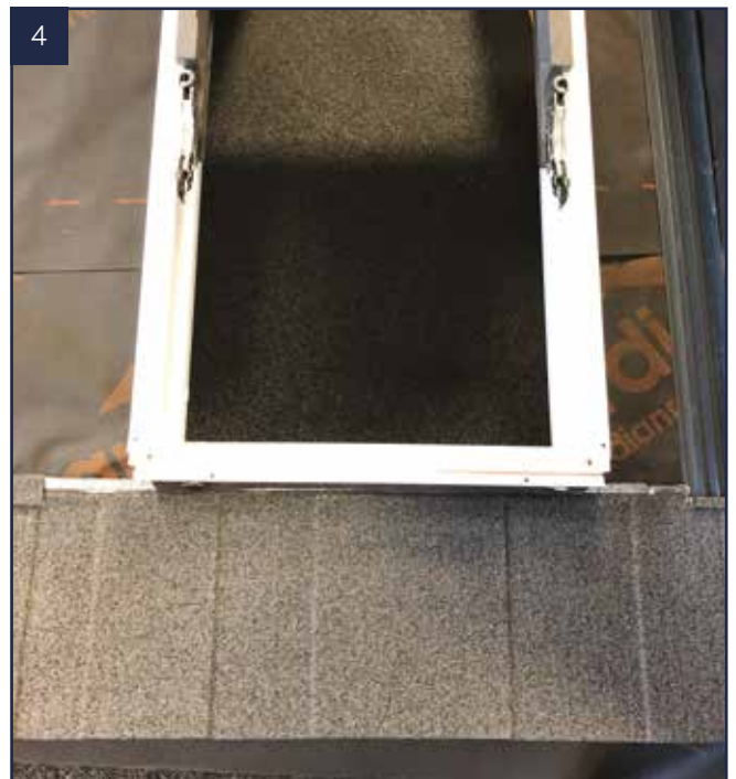
4 Layout of tiles and VELUX® should look be as above.
