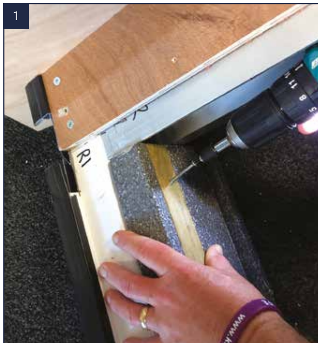
Once the roof has been assembled and the timber has been fitted, fit the eaves insulation.
