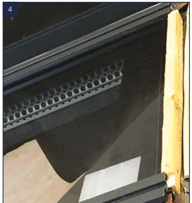
4 Fix the notched timber batten at the top of the solstice panel through into the ridge.
