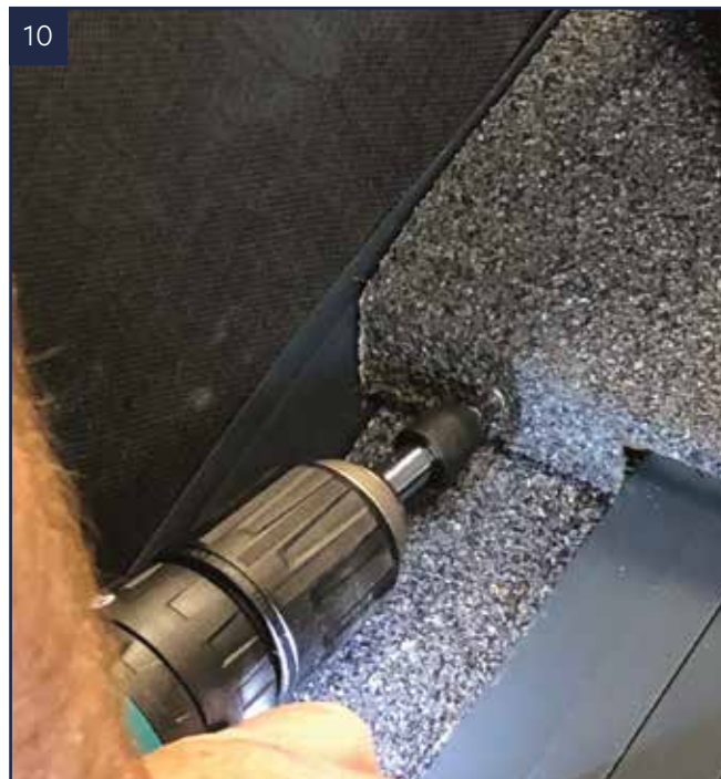
Fix the ridge top cap through into the baton.
