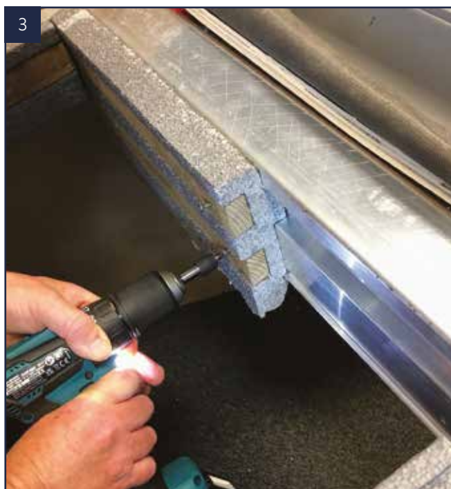
Fit ridge insulation.
