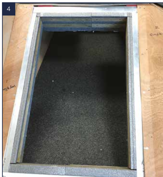
Solstice opening is now fully lined with insulation.
