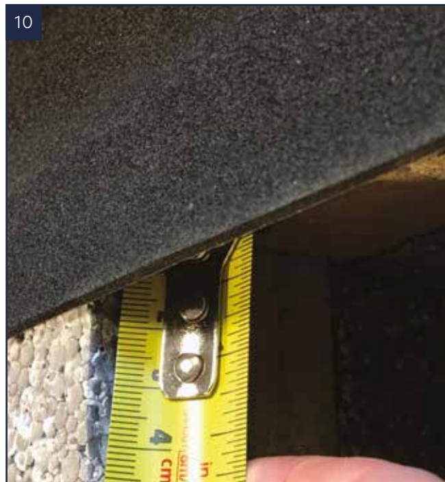
Allow an overhang of 15 mm for the plaster board stop beads.
