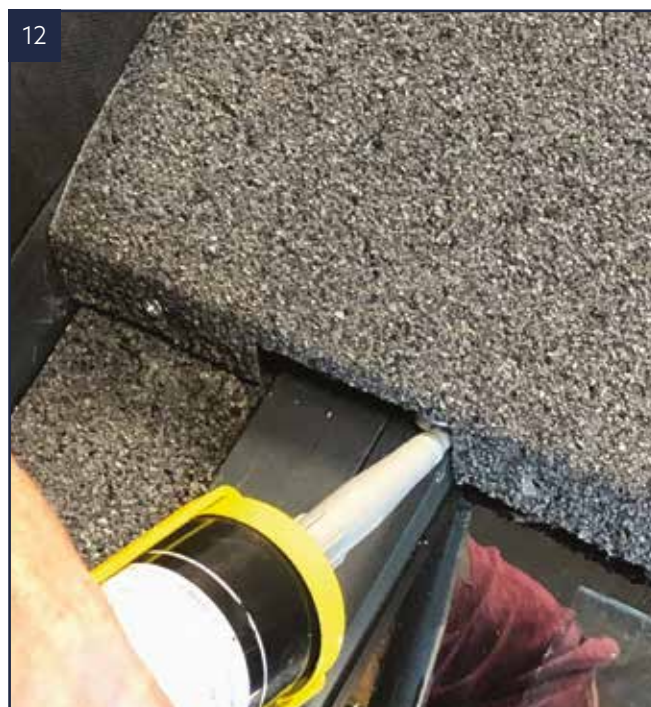
If there is a large gap fill the gap first with silicone allow to start setting.
