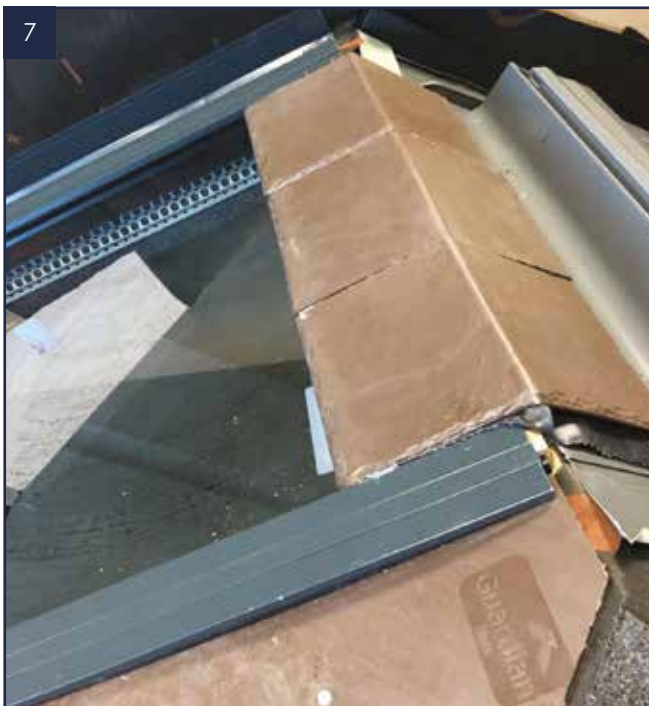
Place a trimmed row of ridge slates over the flashing, these are there for packing purposes only.
