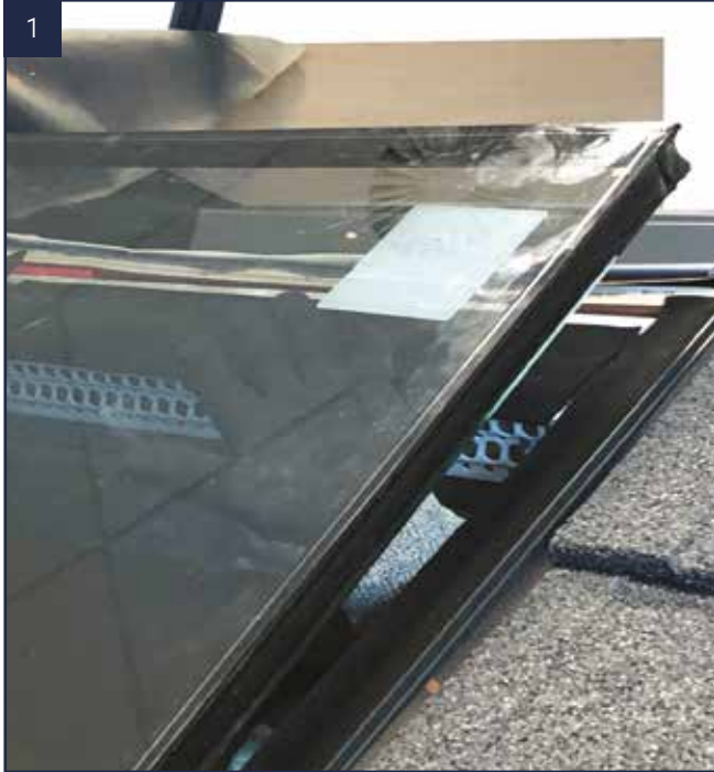
Place glass into position and tile the roof up to the ridge position.
