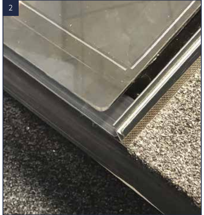
Ensure glass is tight down against the Eaves protector sat onto the foam tape.
