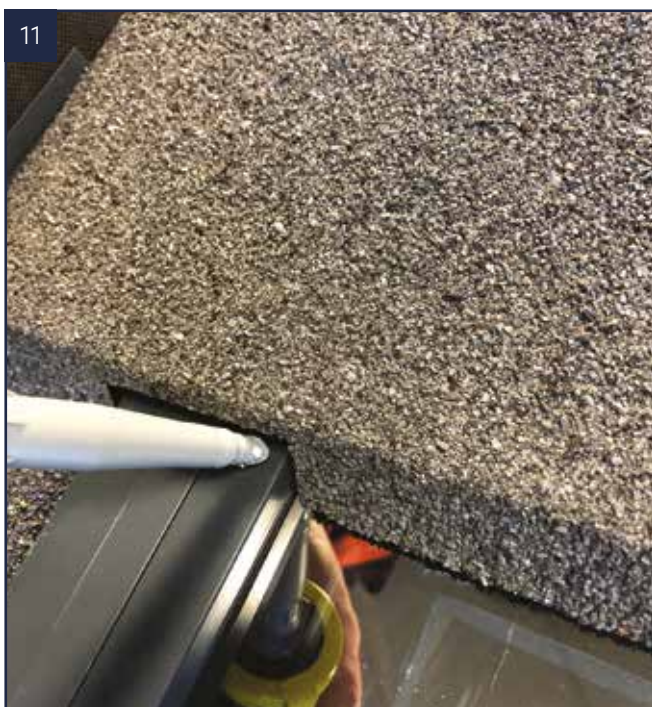
Seal over the top caps against the ridge cap.
