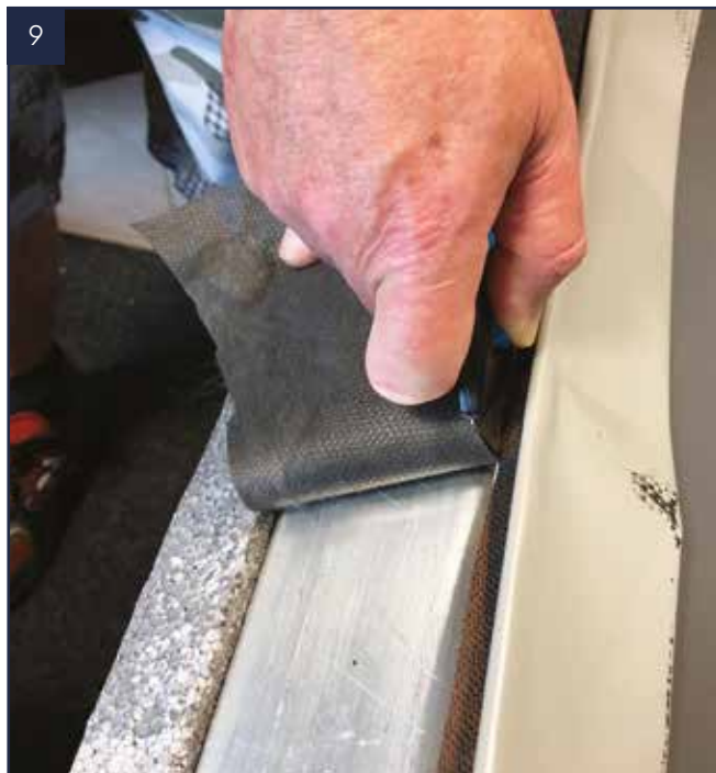
Trim back membrane to expose the aluminium ridge. Apply foam tape to the ridge section.
