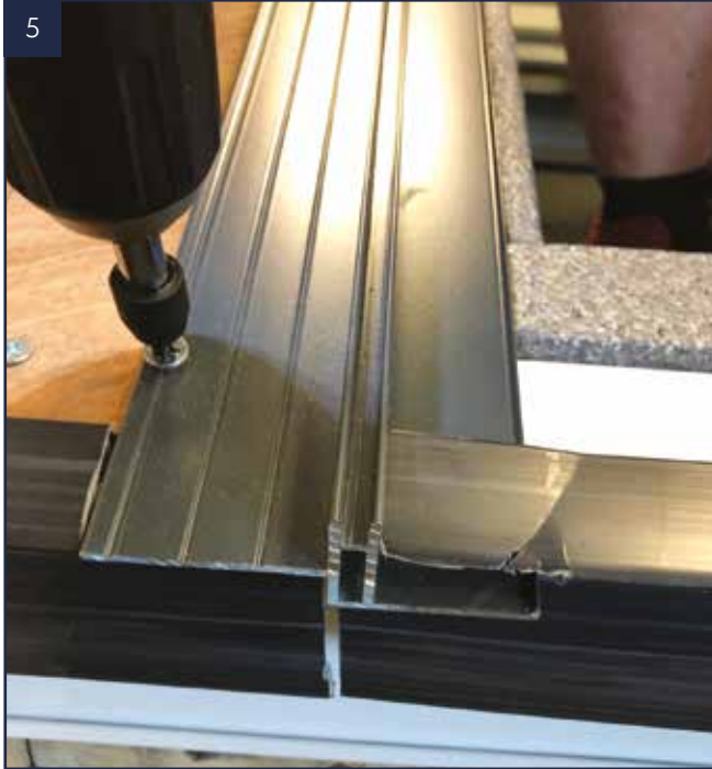
Position solstice bars into place sliding internal side under the eaves protector and up against the timber edge and screw down into place.
