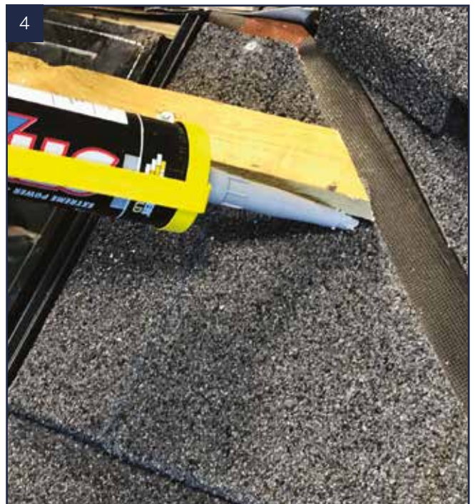
Start sealing along the bottom edge over the tiles.
