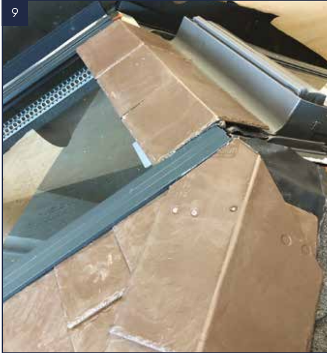
Fit the hip slates starting at the bottom corner of the hips.
