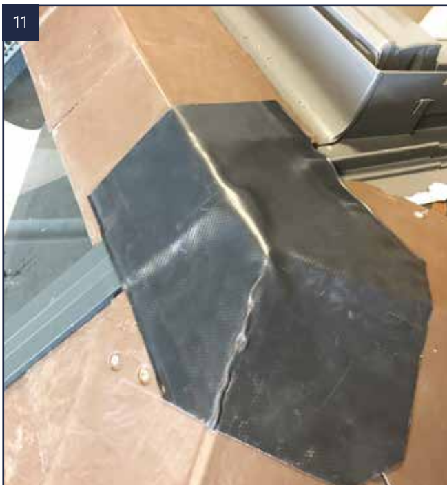
Again with the flashing create an apron detail as above for complete sealing.
