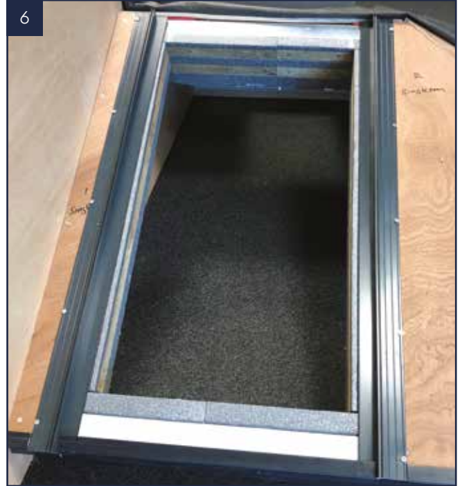
Fixings should be approximately 250 mm apart.
