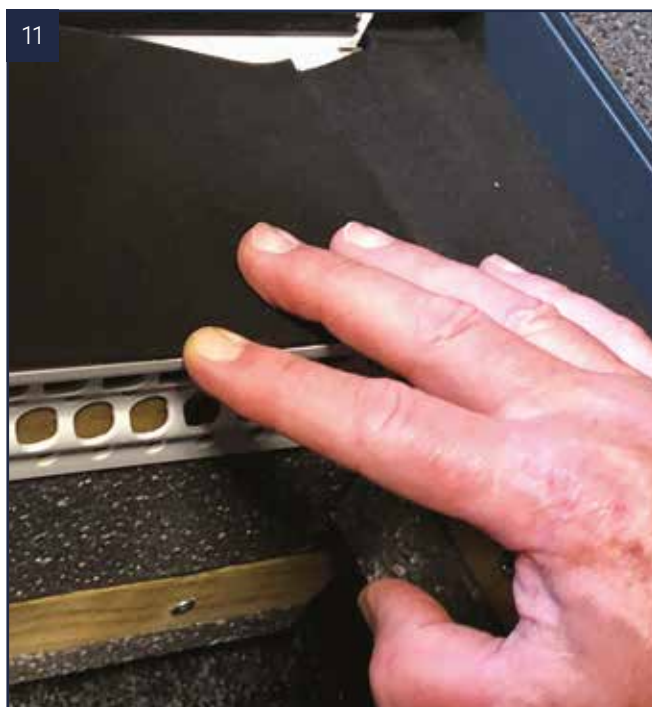
Stop beads can be fitted at this time or after when the internals are being fitted.
