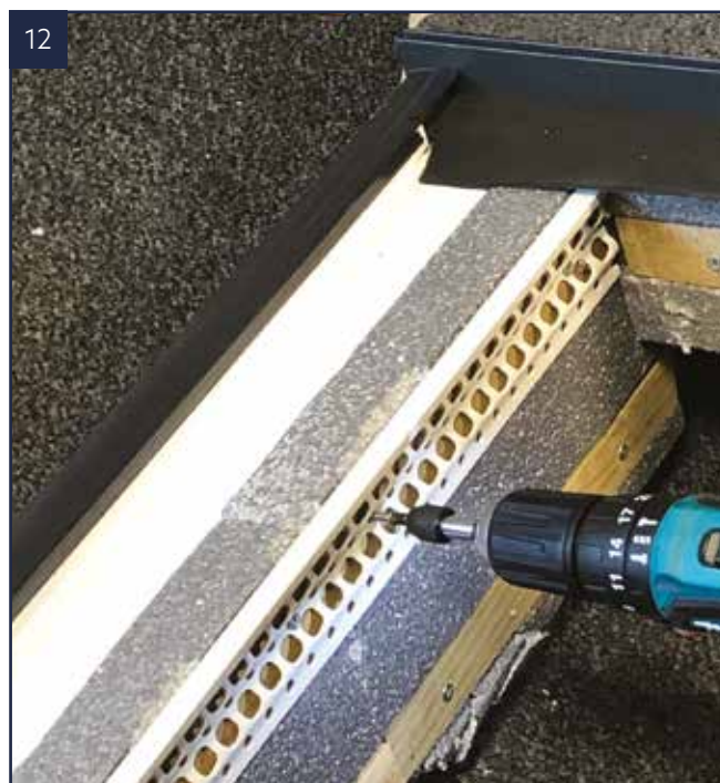
Screw the stop beads into the timber ensuring the top is level with the top of the polystyrene edge.
