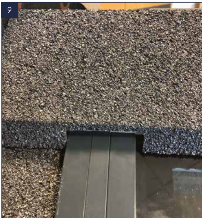
Position pre notched ridge top cap into place ensuring the notches align with the top cap positions.
