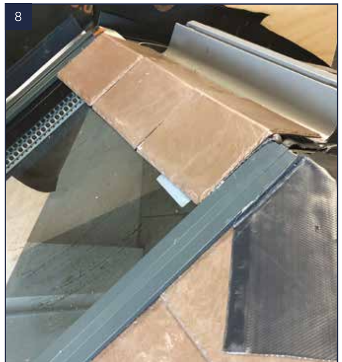
Fit the final top slate into position using the same flashing seal over the top row of tiles.
