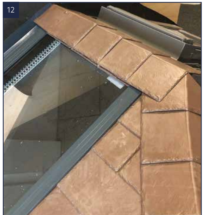
Finally fit the top row of ridge slates fixing down through the slate into the timber batten.
