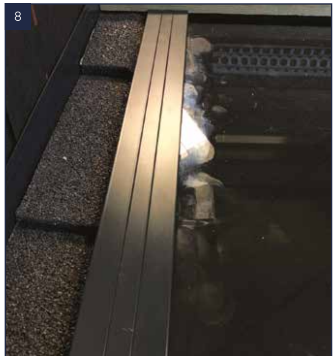
Push fit top cap trim into position.
