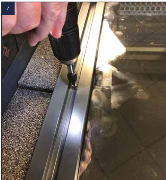
Screw the top caps down into position.
