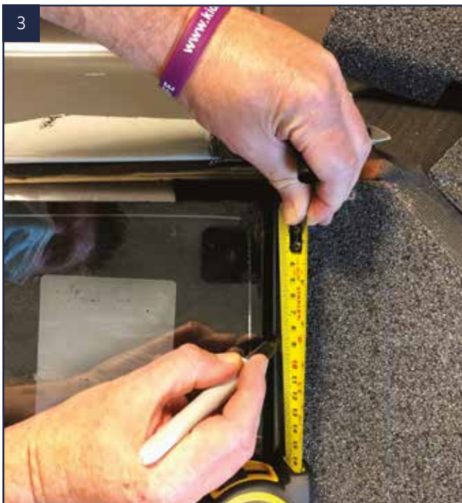
Measure down 85 mm from top of glass for batten bottom edge fixing position, screw batten down at each end.
