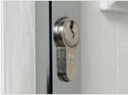
Ultra high-security cylinder lock
